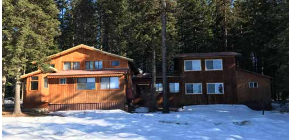
The original home built by Jeff Reich and his family (left section), is now Laymen Ministries' main office, with additions for bookstore, print room, and office space.
